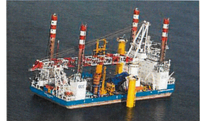
Fredrich Ernestine installing a transition piece
