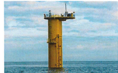
Foundation Installed at Gwynt Y Môr
